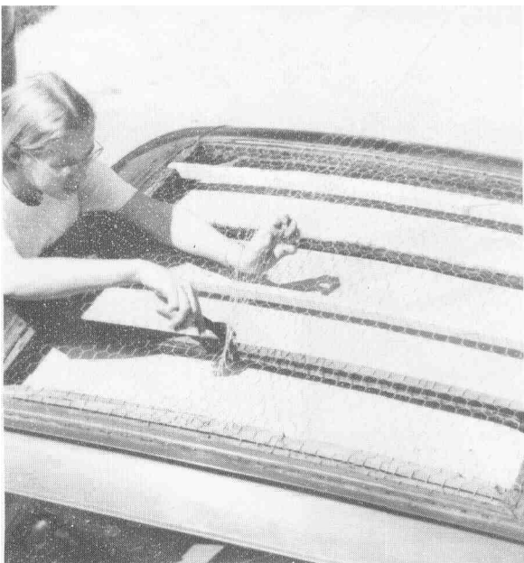
Installation of chicken wire.
